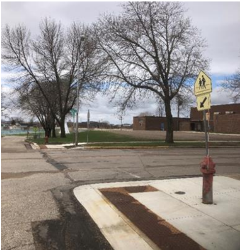
Figure 4: Chippewa Co. Rd 2 and 4 th Avenue NE
